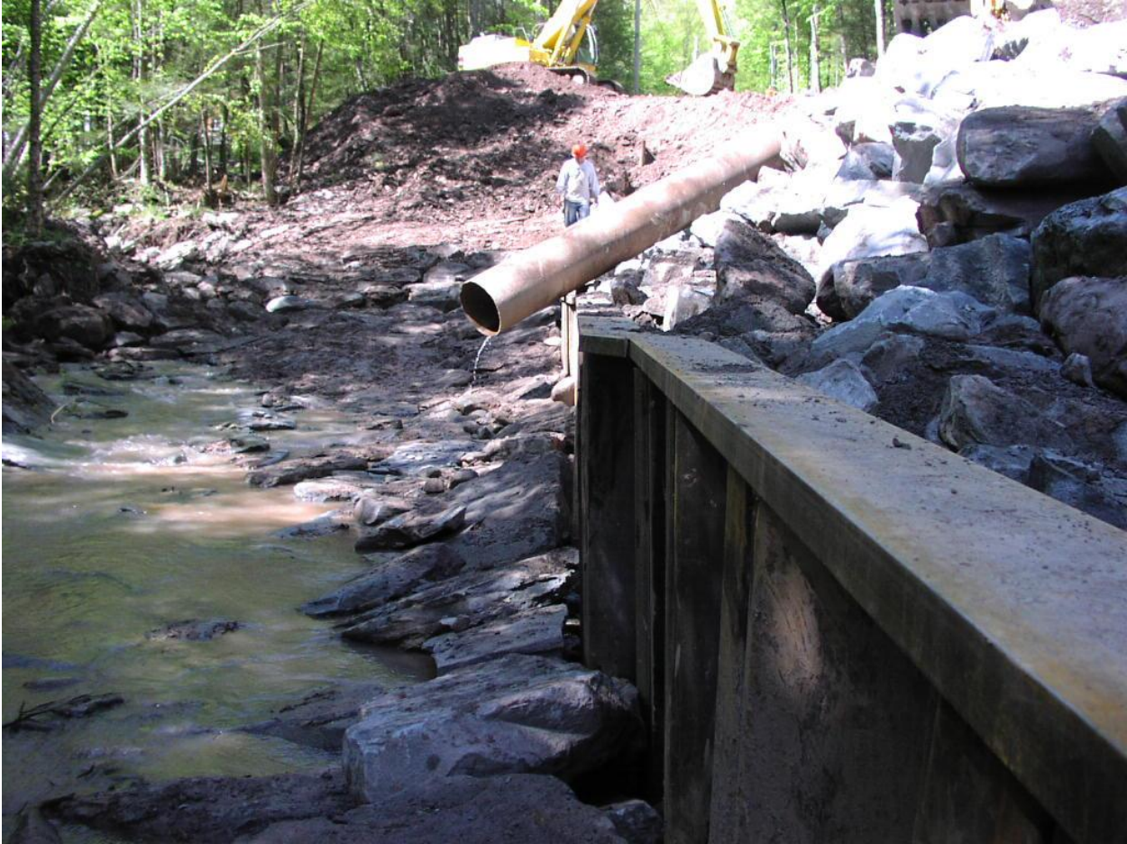
Completed Sheet Piling
