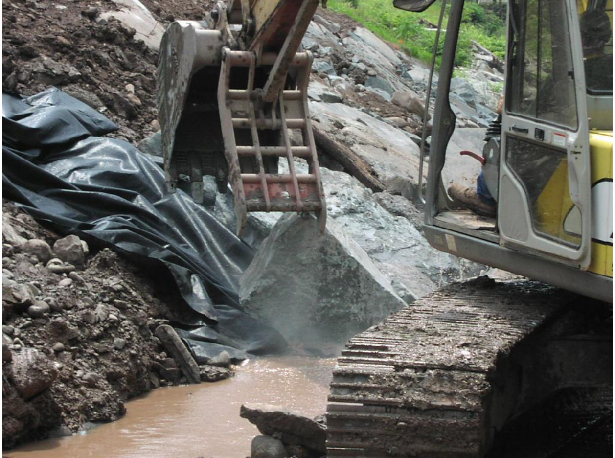
Placing stone in key trench.
