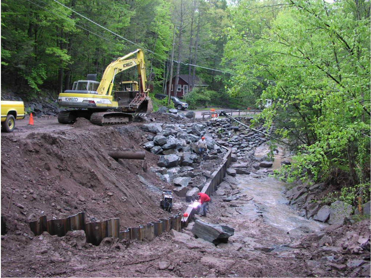
Welding Sheet Piling
