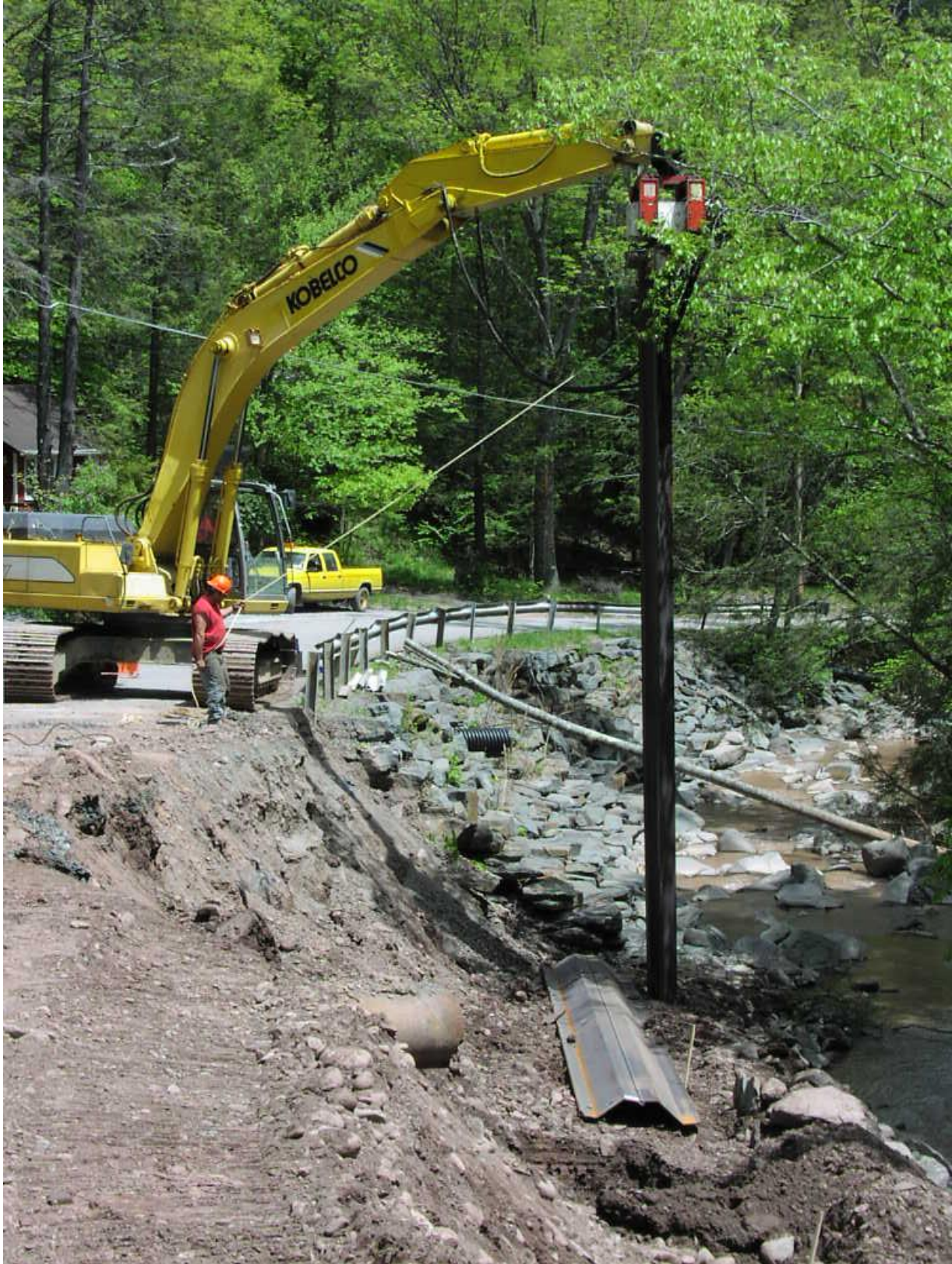
Driving Sheet Piling
