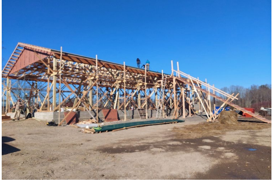
Construction of covered barnyard agricultural best management practice fall 2023
