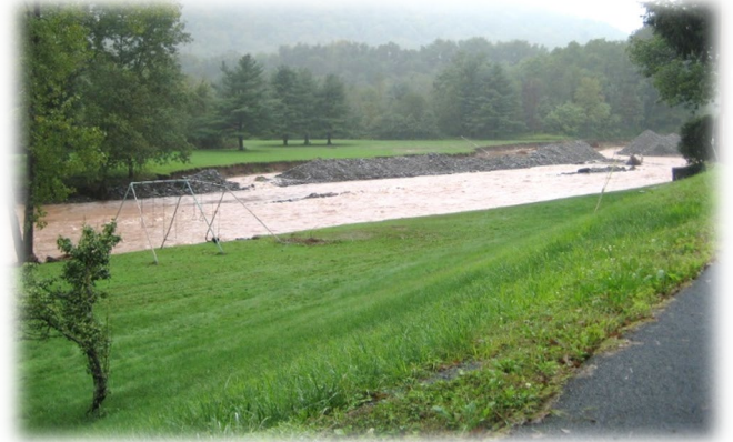
Degraded Riparian Buffer near Shandaken, NY. Turf lawns provide no bank stability and offer little ecological value to stream corridors.
