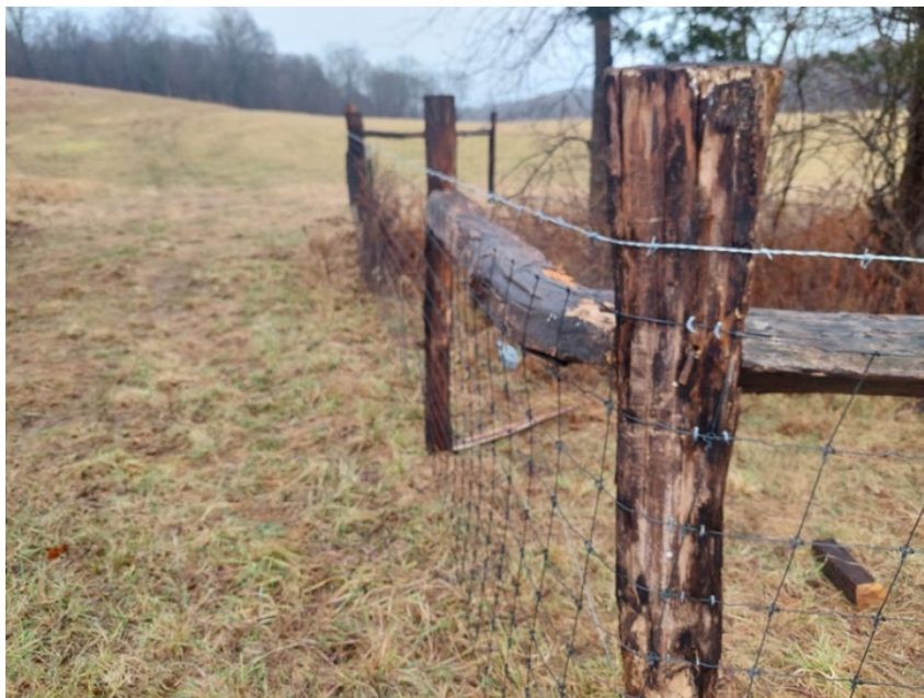
Completed fence for rotational grazing system
