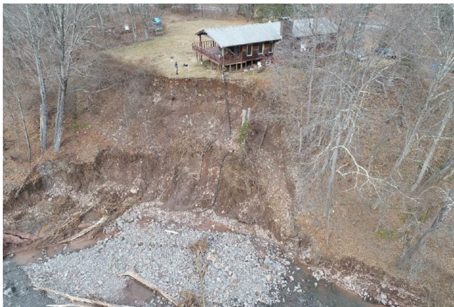
Hillslope failure and bank erosion (left photo) and stabilized hillslope and stream channel realignment (right photo) at Stony Clove Creek restoration site.
